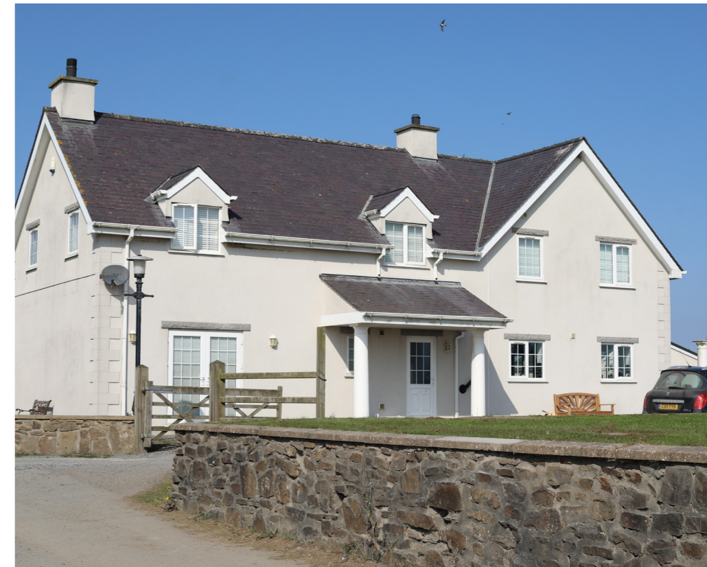
View of eastern facing (entrance) aspect of dwelling
