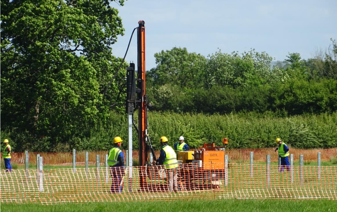
Insert 6: Inserting a Stanchion
