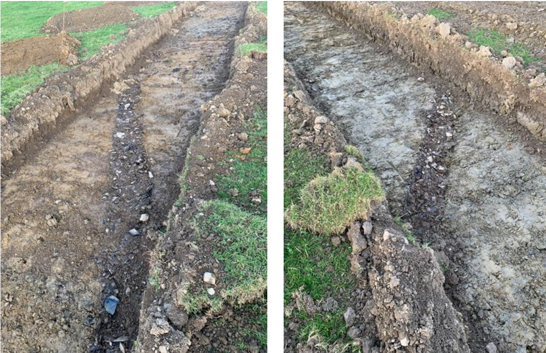
Inserts 64 and 65: Shale Drains at Tan Rallt
