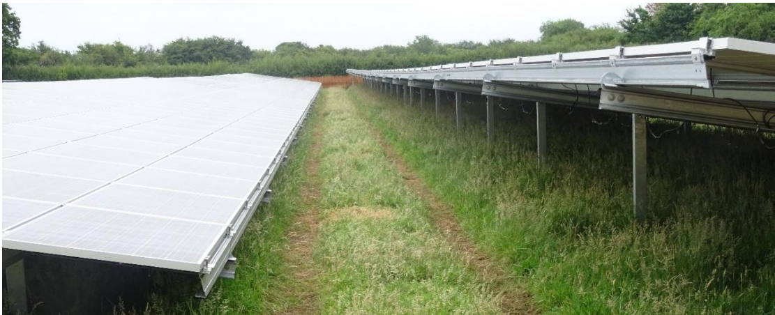
Insert 13: Following the Bolting-on of the Panels
