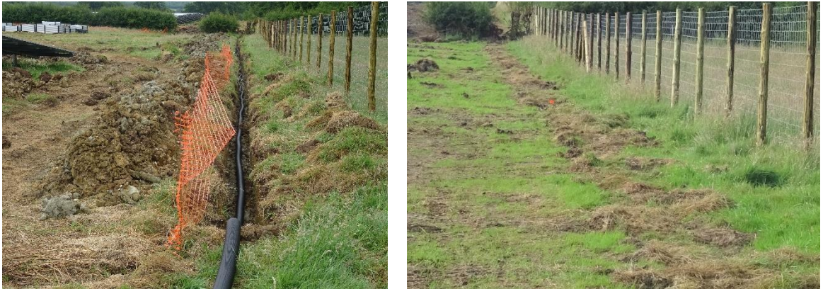
Inserts 19 and 20: Example of Cabling Being Installed
