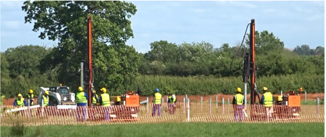
Insert 7: Team Installing Panels
