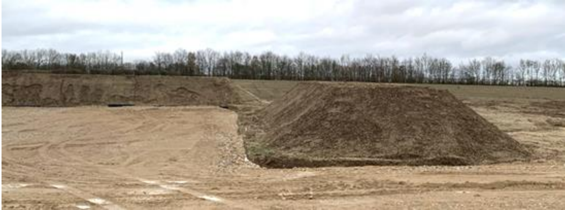
Insert 26: Example Topsoil Storage Bund
