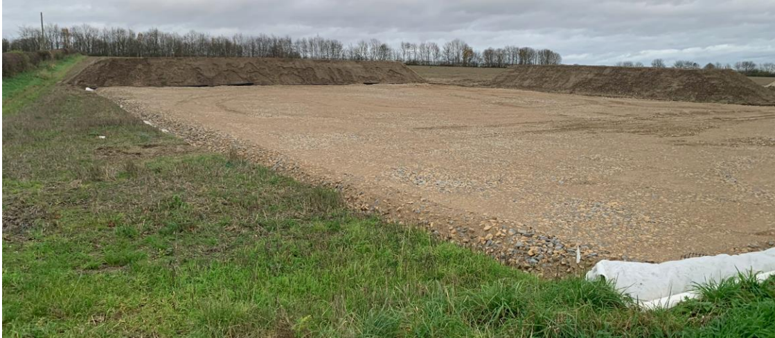
Insert 24: Newly-laid Construction Compound (Elsham-Lincoln Pipeline)
