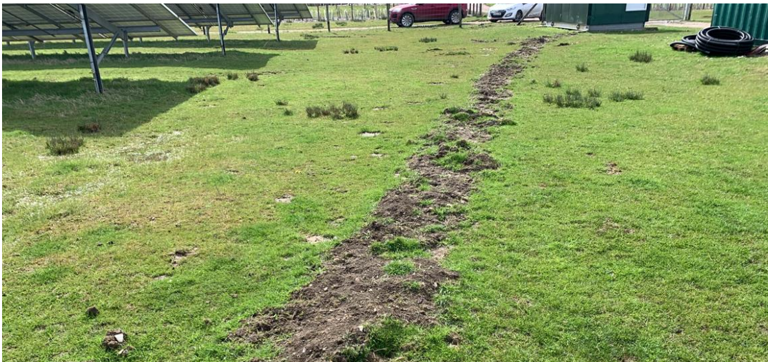
Insert 34: Trench During Wet Period
