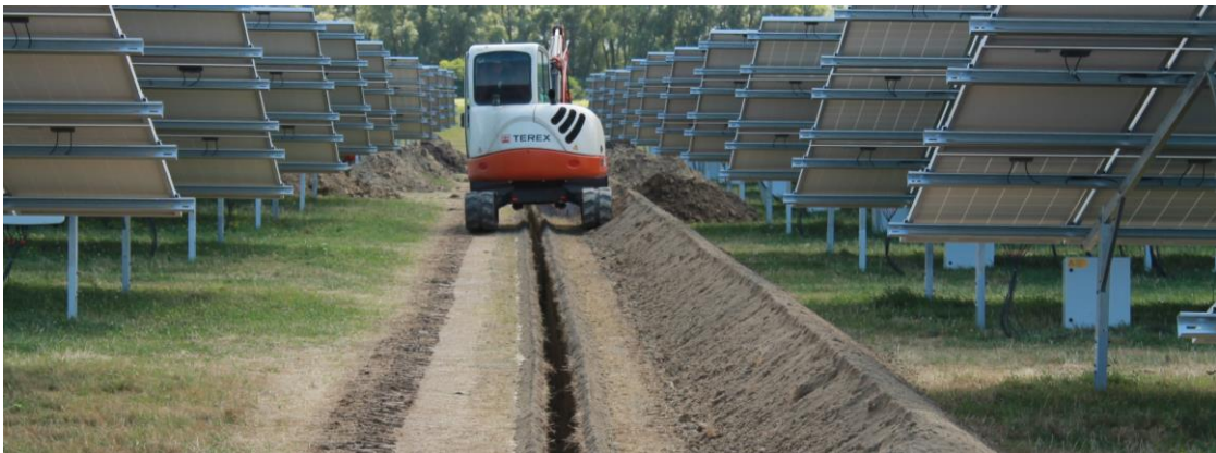
Insert 21: Cable Trenching, Central Row
