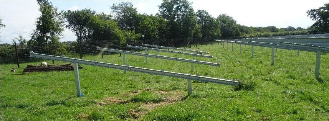
Insert 9: Legs being Installed (this at Tiln Farm, Retford, January 2023)
