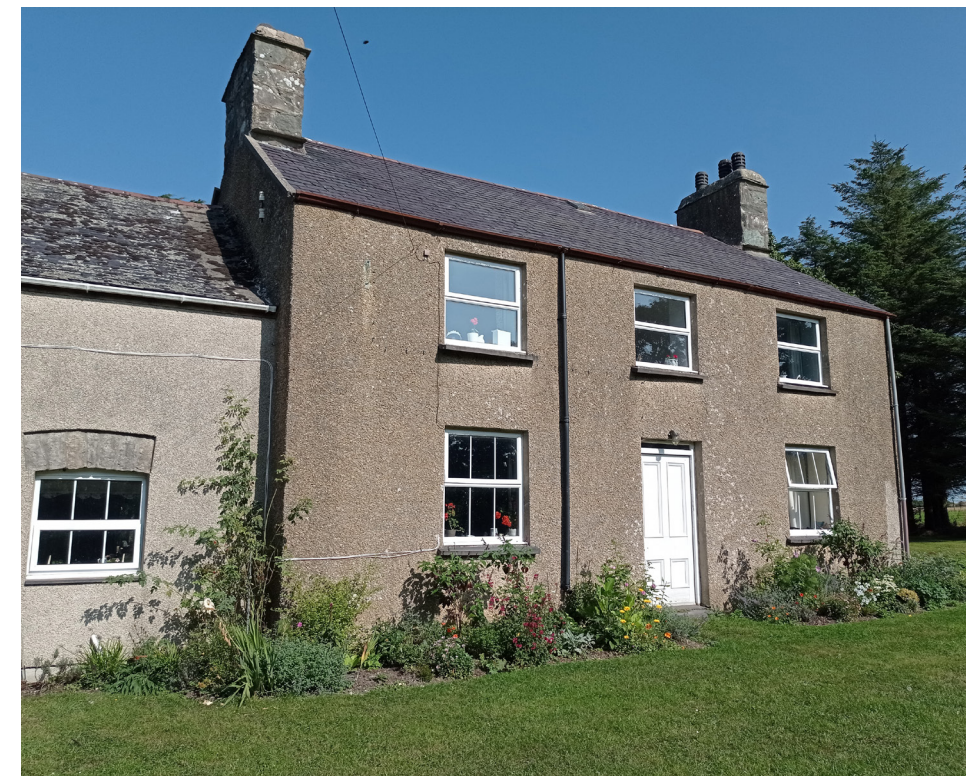
View of north eastern facing (entrance) aspect of dwelling
