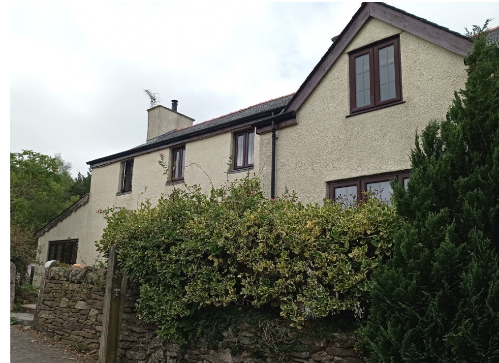
View of north east facing (main entrance) aspect of property
