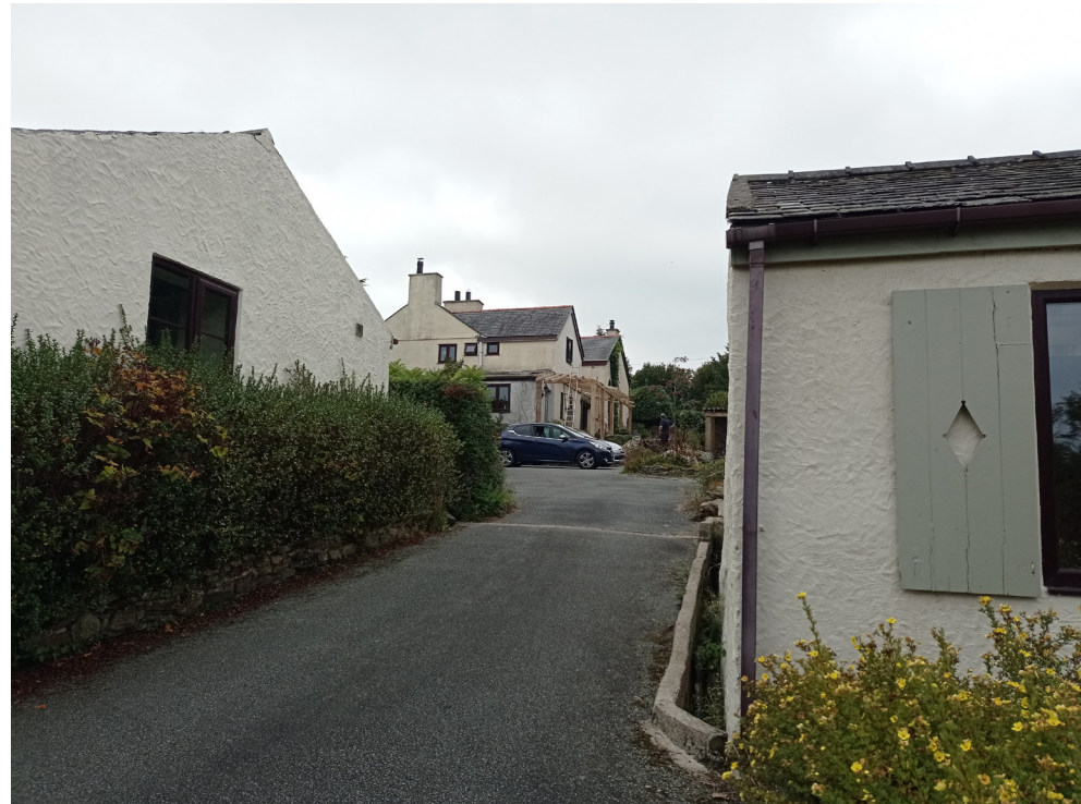
View of north northeast facing aspect of main dwelling
