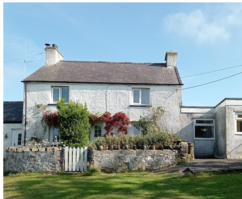
View of north western facing (entrance) aspect of the property
