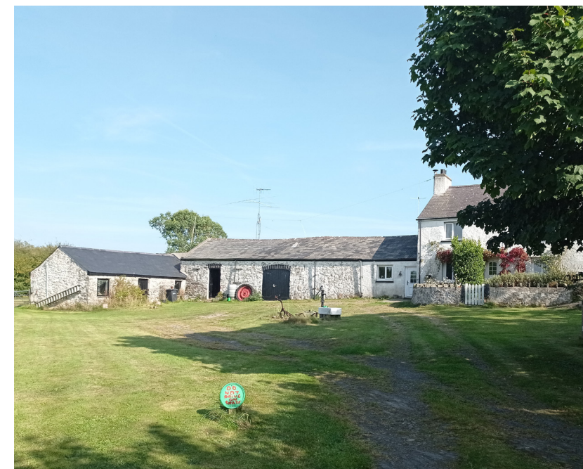
View of north western facing aspect of the property
