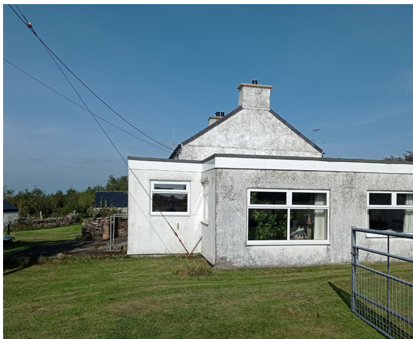
View of south western facing (extension) aspect of the property
