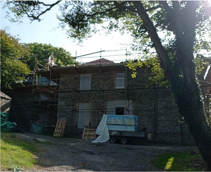
North west facing aspect of dwelling under construction
