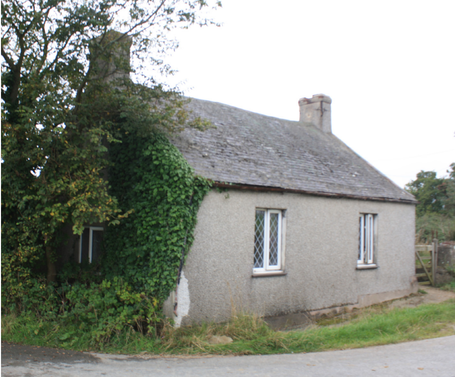
View to show north west facing aspect (frontage) of dwelling
